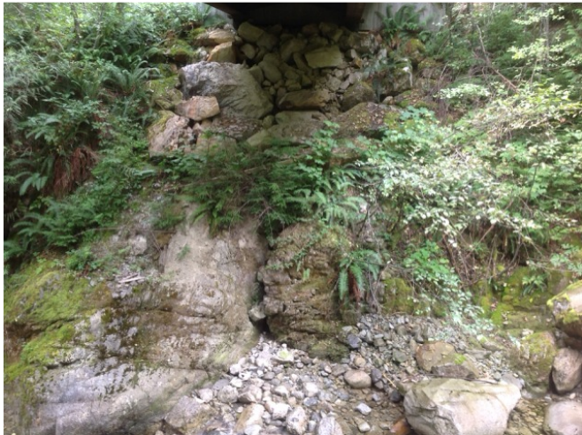
Right Bank Abutment when facing downstream
