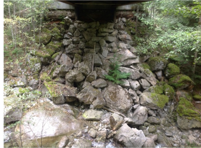
Left Bank Abutment when facing downstream
