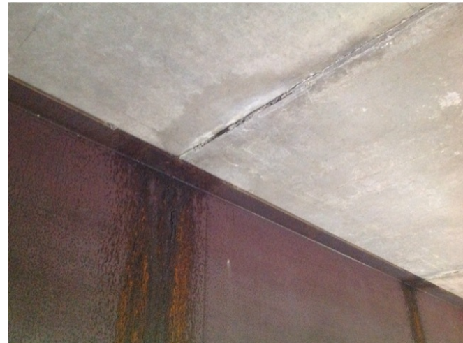
Deck joints from below
